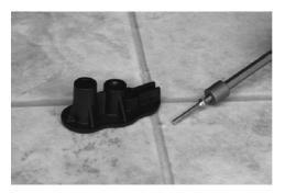
The screw is now set 1/5 of an inch below the floor. Take a hammer and tap the small bump that is left to smooth out the hole and force the hole to fill over.
