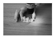
Pre-drill a hole in the floor with a 1/8 inch drill bit down 2 1/4 inches.
