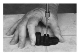
Once you find the joists, focus on the spot on the joist where the movement and squeaks are coming from. Then drive the screw through the shorter opening in the fixture.
