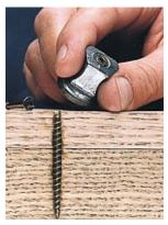
The best way to determine bit size is to try it on an inconspicuous part of the flooring (perhaps inside a closet) and drive the screw down through the fixture. The screw should snap just as the head hits the fixture. If it does, you can use it on the rest of the floor. If it doesn't, then drop down a size on the drill bit to put more pressure on the screw.
